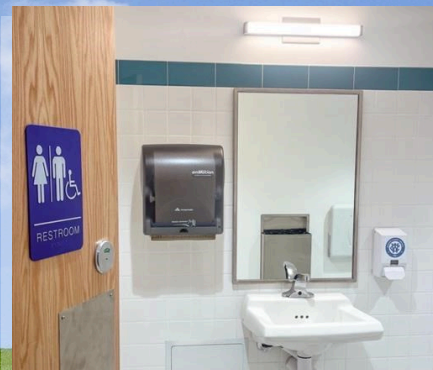
New family restrooms were constructed in the Young People's Library on the main level of the Downtown Reno Library in 2023.
