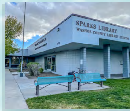
The newly remodeled Sparks Library has been at its current location since 1964.
